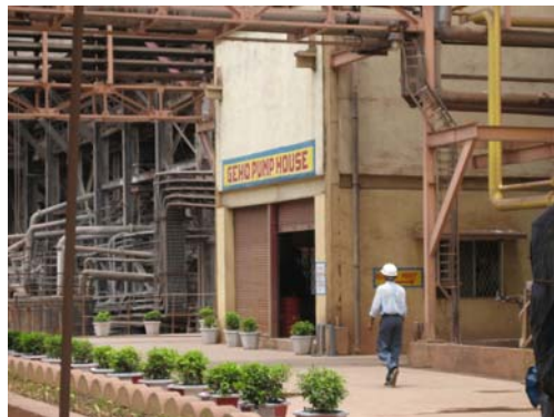
Geho pump house at the Hindalco site.
