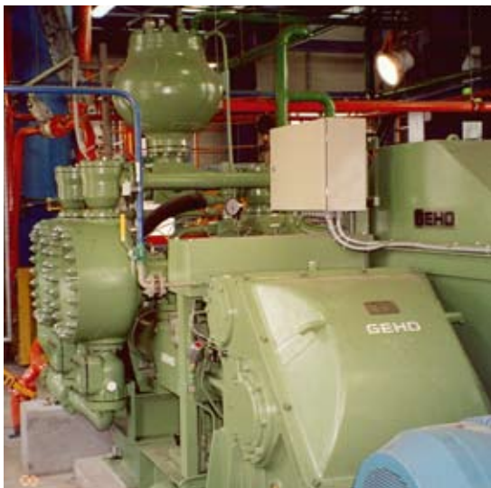
Geho duplex piston diaphragm pump at the Timisoara Power Station, Romania, handling fly ash and slag slurry.
