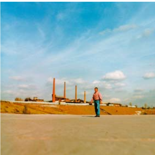
The Elektrarna Ledvice Power Plant deposits residue from coal combustion and flue gas desulphurisation at a distance of 4700 metres against the slopes of an abandoned open pit.
