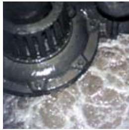
Below: Floor clean-up sump pump
