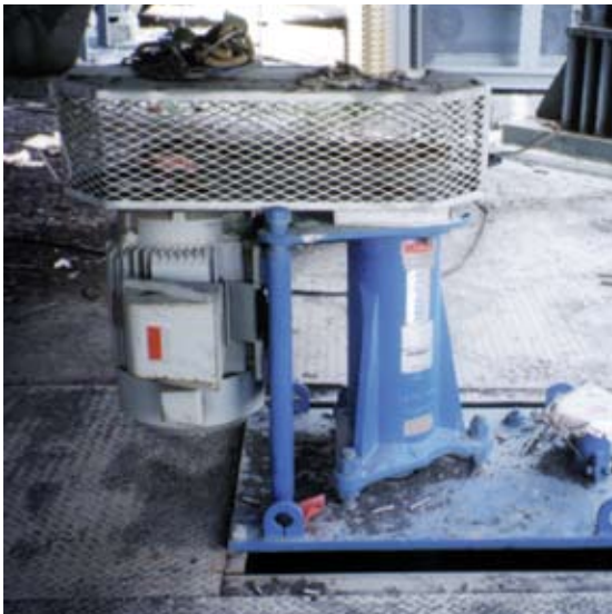
Below: Floor clean-up sump pump
