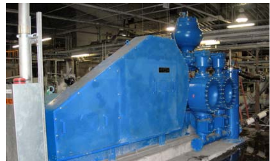
GEHO® piston diaphragm pump, model ZPM 700, for high density fly ash disposal.
