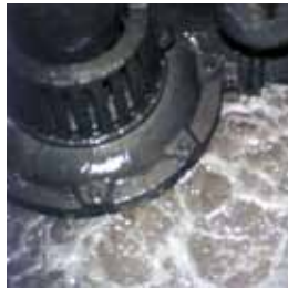
Below: Floor clean-up sump pump
