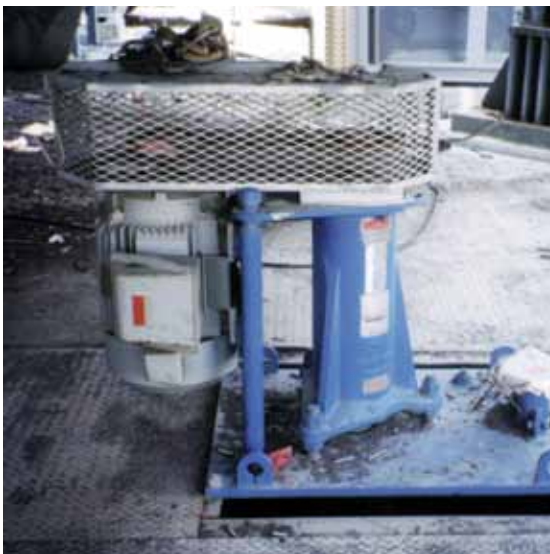
Below: Floor clean-up sump pump
