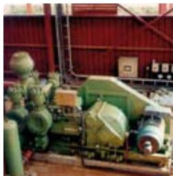
Red mud and sand transportation, Alcoa San Ciprian, Spain
