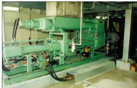
Hyougo, Japan: sewage sludge transfer
