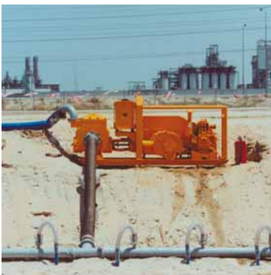
Bottom left: Dewatering of construction sites at home and abroad
