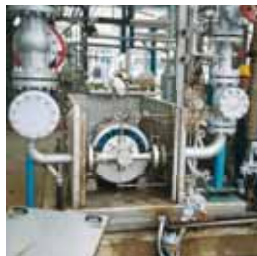
Top left: The Netherlands, propeller pumps for brine circulation
