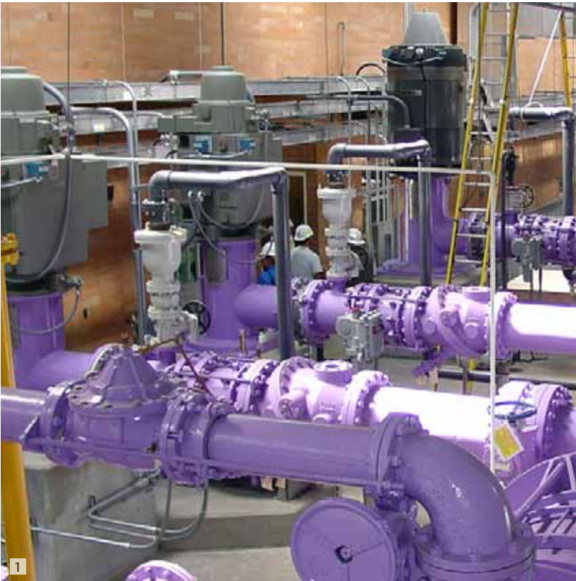
1: Water re-use pumps 2: Field installation 3: Booster pumps
