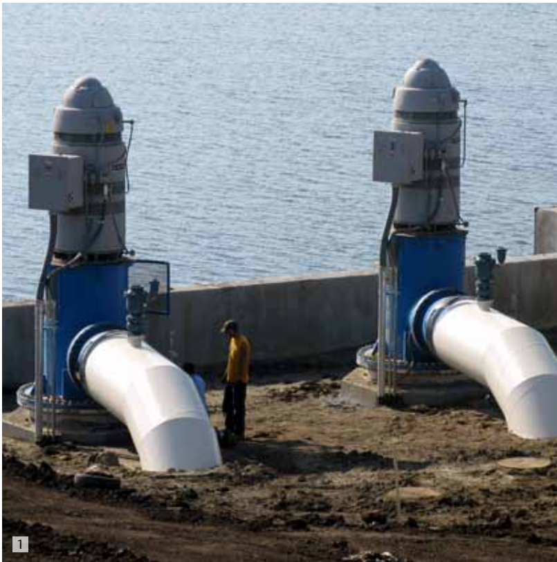
1: Raw water service pumps 2: Water pumps
